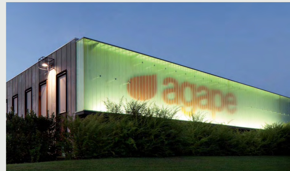
Sede operativa Agape / Agape headquarters building
