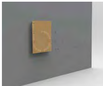
5. Attachment of letter b on wall pins.
